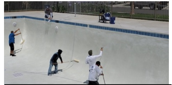
MicroGlass Application on New Commercial White Plaster Finish
