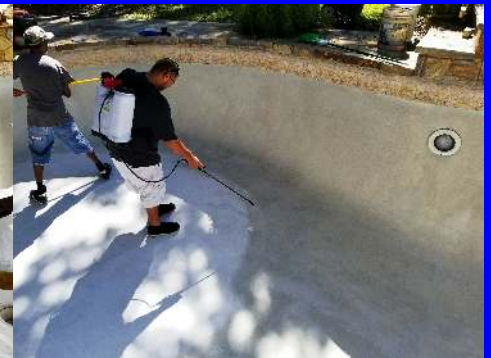
Here you can see the results of spraying and back rolling.
