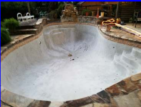
Curing overnight after spraying
