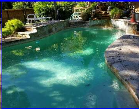
After filling with iron contaminated well water.
