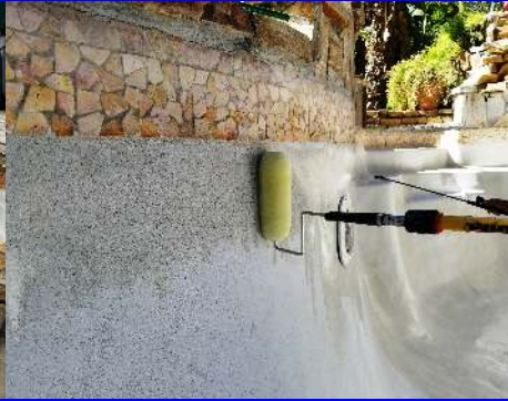
Spraying Microglass & back rolling with a dry 1 1/2" roller cover.
