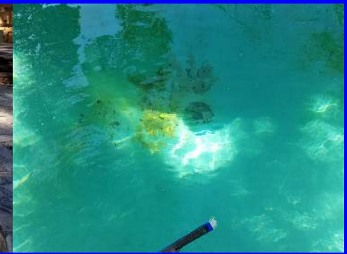
Iron deposits in pool which did not stain or adhere to pool surface.
