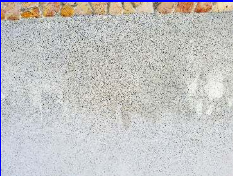
Here the Microglass has been sprayed on the wall.
